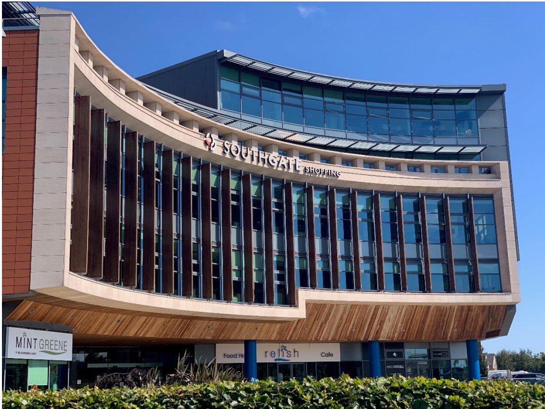
Figure 2.2: View of Southgate Centre
